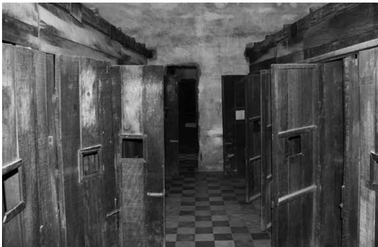
Single cells in the torture prison S-21. Some 14,000 to 20,000 Cambodians were incarcerated in the former school complex between 1975 and 1979. | Source: © Maximilian Jürgens.
